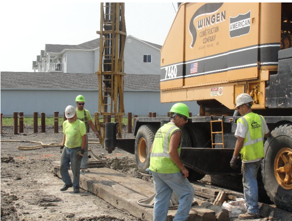
Fargo Water Tower Piling
